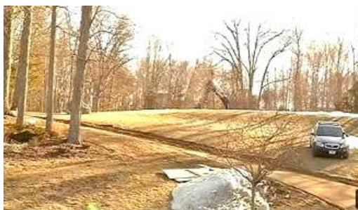
Nancy Lanza's house is razed to the ground, allegedly because it makes people feel bad. The demolition firm did the work pro bono, hence no need for open bidding, Photo: CBS News
